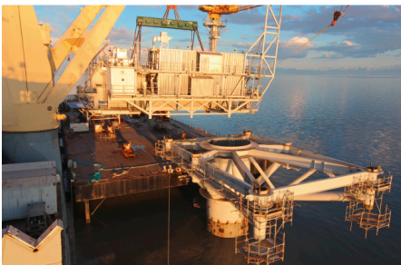
Work in progress: installation of the Topside
