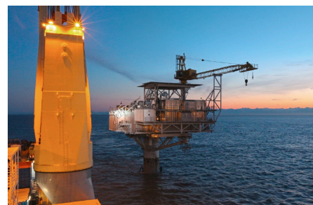
Mission accomplished: whole production platform completed
