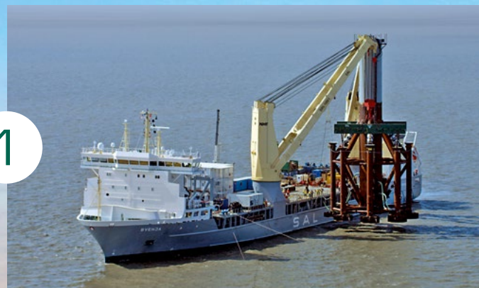
Subsea installation of Monopod
