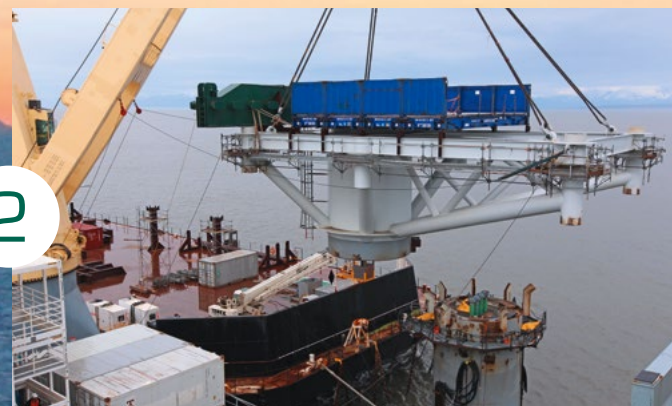
Installation of Modular Support Frame (MSF)
