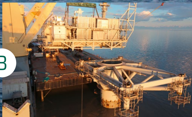
Installation of Topside
