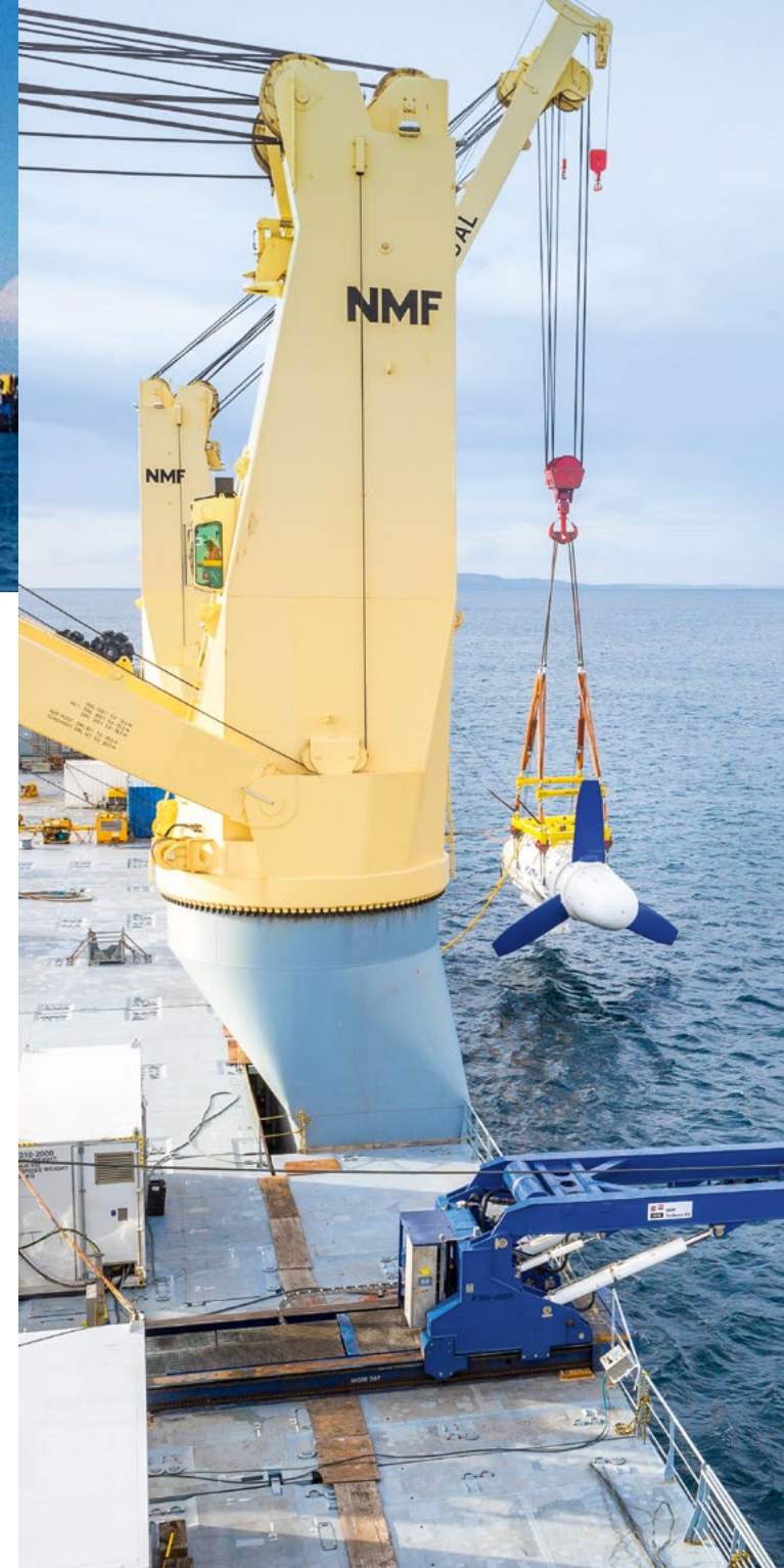
Installation of subsea platform (1 000 t)
